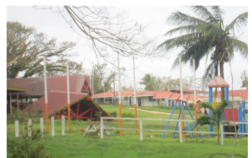
Dislodged roof on Independence Park
